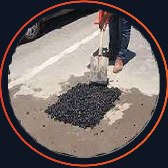
Fix Cold Asphalt
